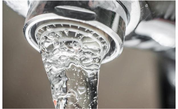
When considering replacing bathroom faucets, check the flow rate of your current fixture by examining the tip of the faucet head. Older faucets typically have higher flow rates, so consider replacement or adding an aerator.
